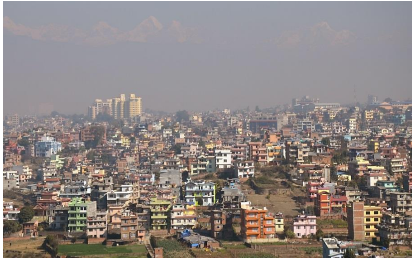
Figure 3-23 Development on hillocks surrounding KV
