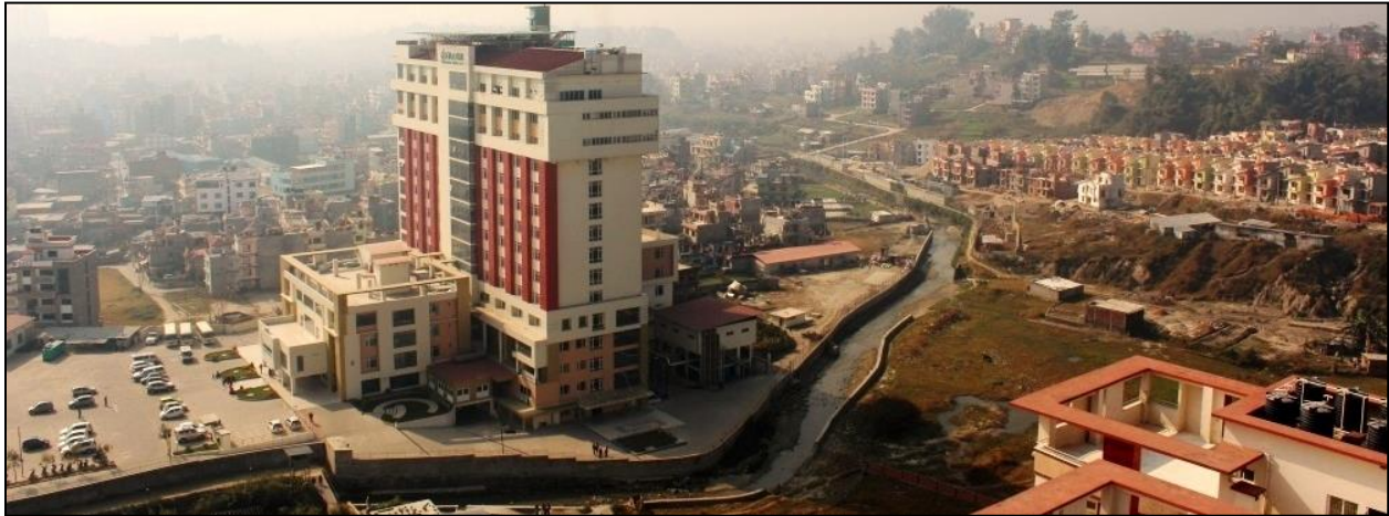
Figure 1-12 Large buildings for apartments, hotels, hospitals and other commercial use is a relatively new phenomenon after the relaxation on multi-storey building permits and the political instability
