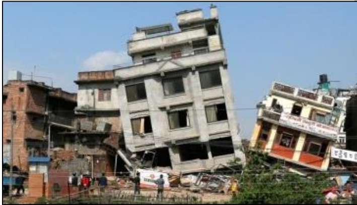
Figure 1-6 Damaged buildings in Kathmandu lean to their sides due to April 25 earthquake in Sitapaila Image Source: KVDA
